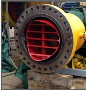
Pigging bar insertion plug installed into hot tap penetration
