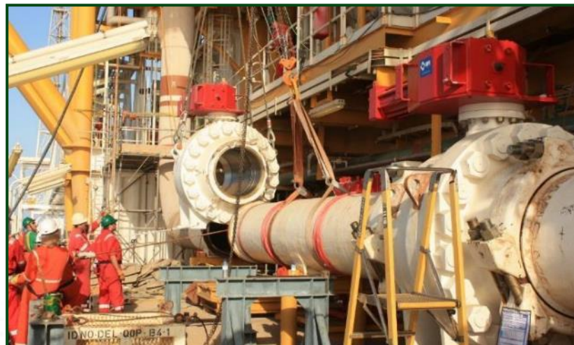
36" Valve Replacement and Repair – Pipeline Remains Pressurised
