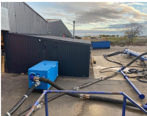
Figure 11: Water Testing Set Up
