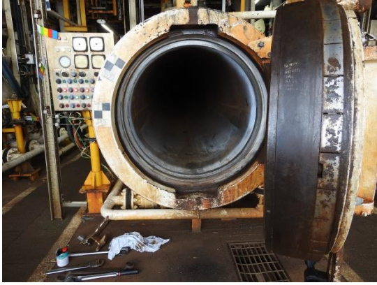
Figure-1 Launcher and Closure Door
