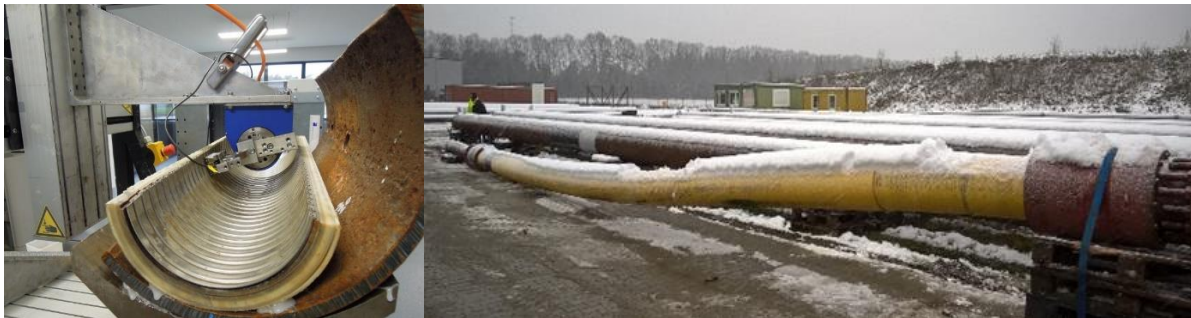
Figure 4: Flexible Pipe Pull Through and Lab Test Setups
